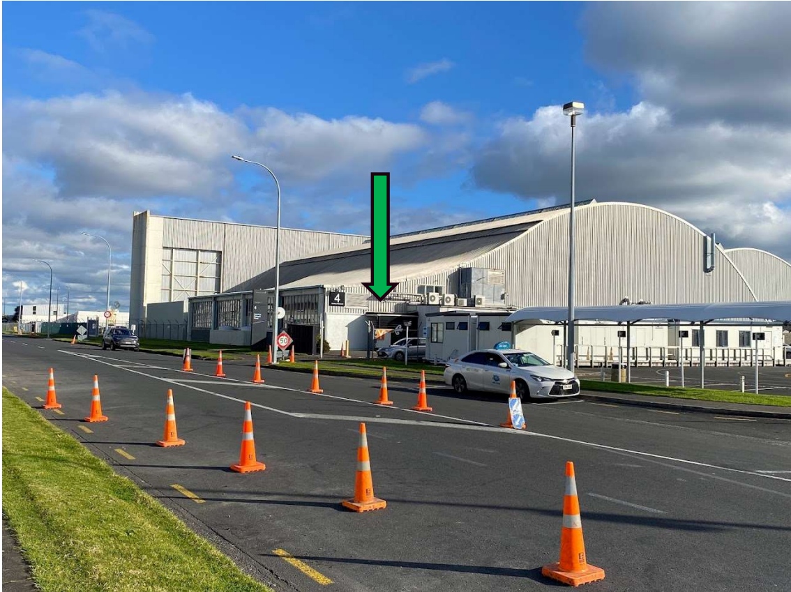
FIGURE 1: MAURI ROOM ENTRANCE
